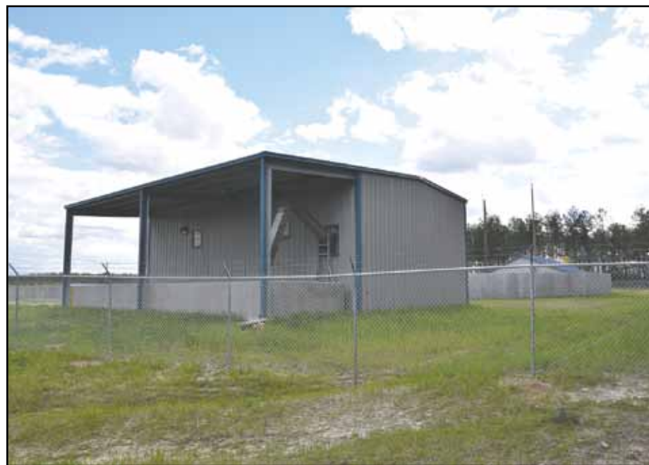
Now open: the wastewater treatment plant.
